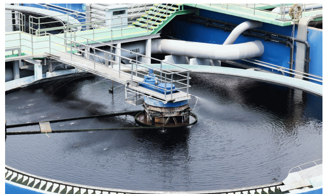
Wastewater treatment is another industry where gas detection is commonly used
